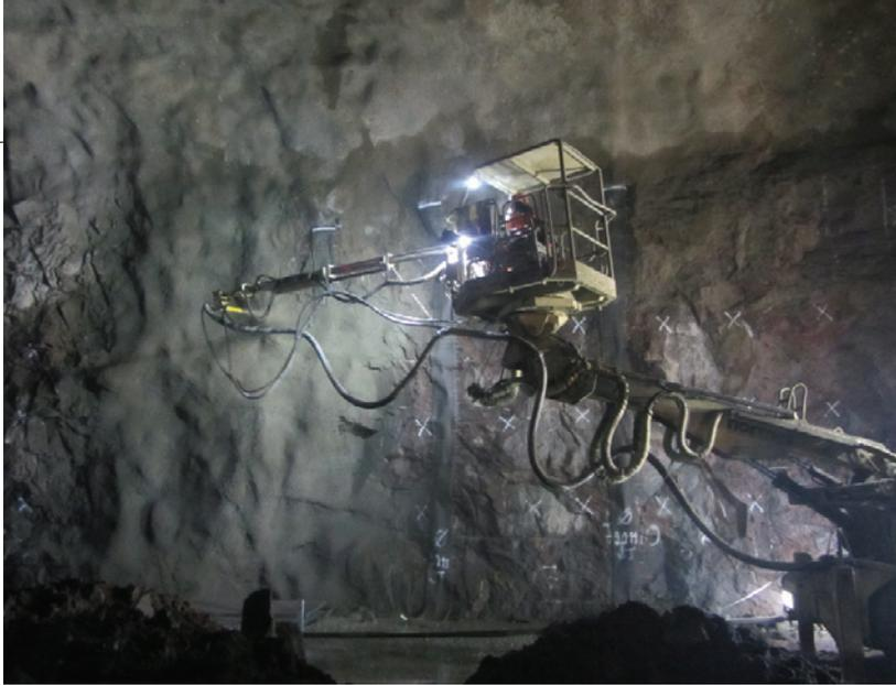
**Left: Spraying of MSFRS at the Helsinki West Metro Extension project**
