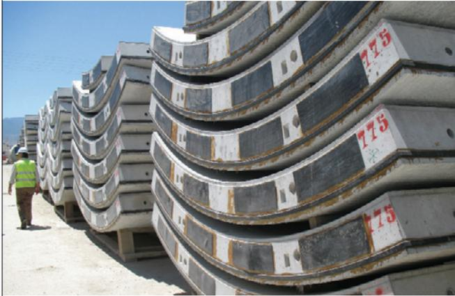
**Above: Malaga Airport High Speed Rail segmental lining used a combination of steel cage and macro-synthetic fibre reinforcement**
